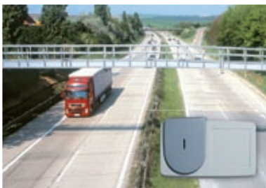
Mautsystem (tolling system)
