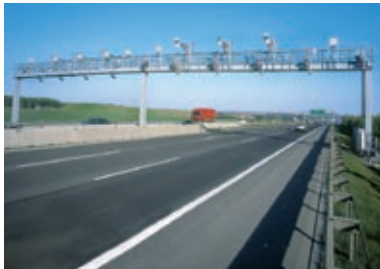
Road Solution Projects (RSP)
